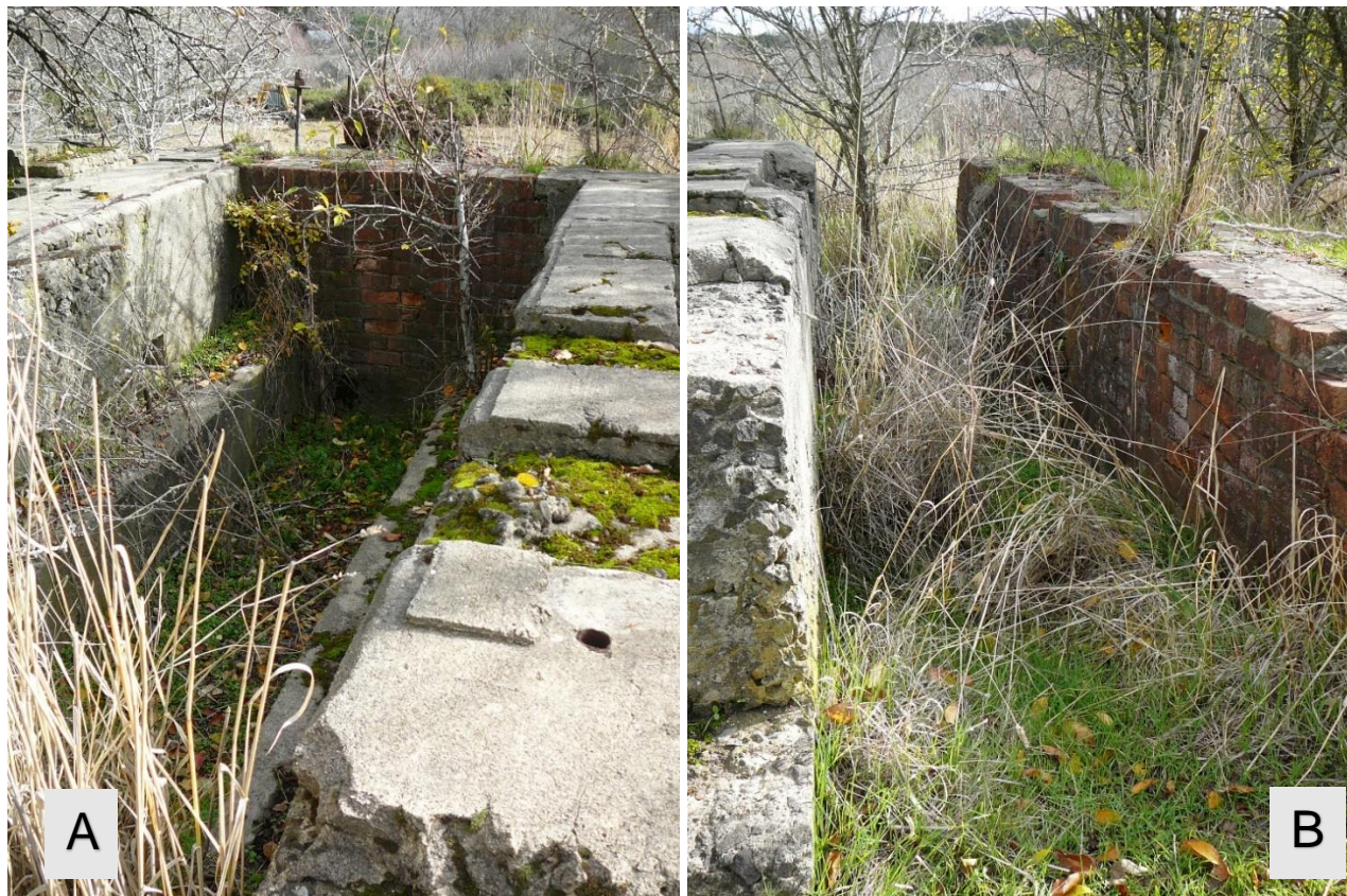
Figure 41. The concrete U-shaped engine bed (A) and adjoining brick wall (B)
